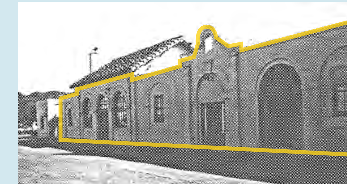
West Facade | Fachada Oeste
