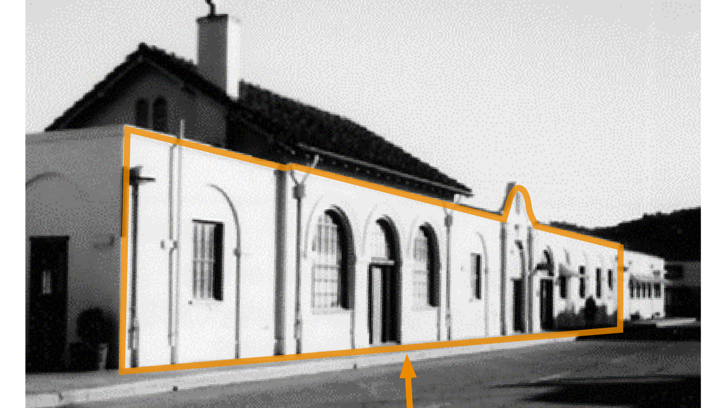
West Facade | Fachada Oeste
